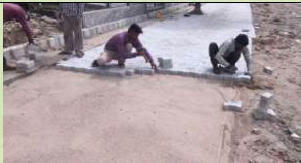
Tile work on 120 ft Road Model Town in progress
