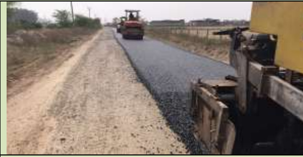
Bitumen work in progress on Jamshar Diary Road
